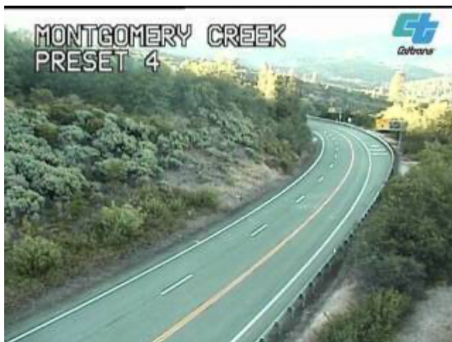
Figure 86. Highway 299 in the mountains between Montgomery Creek and Burney. Highway 299 is two lanes, with some three-lane passing sections, and is the only viable evacuation route out of communities like Burney, Montgomery Creek, and Round Mountain. Source: Caltrans 2021b.
