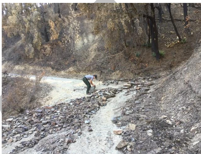
Figure 8. Following the Carr Fire, accelerated erosion of burned slopes on Shasta Bally began depositing large amounts of debris on Mill Creek Road in the Whiskeytown National Recreation Area. Source: NPS 2021.
