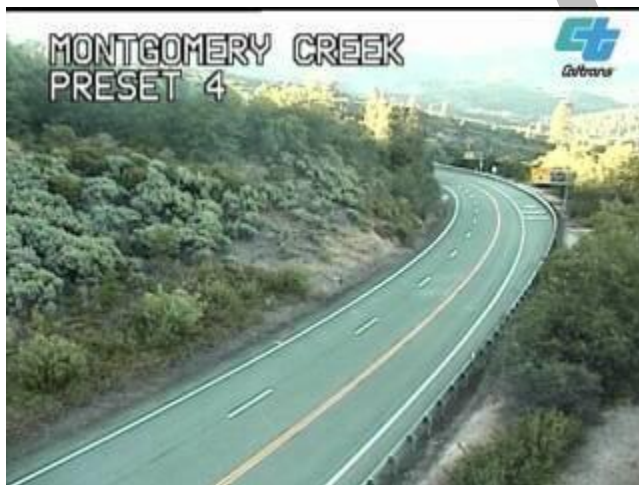
Figure 3. Highway 299 in the mountains between Montgomery Creek and Burney. Highway 299 is two lanes, with some three-lane passing sections, and is the only viable evacuation route out of communities like Burney, Montgomery Creek, and Round Mountain. Source: Caltrans 2021b.
