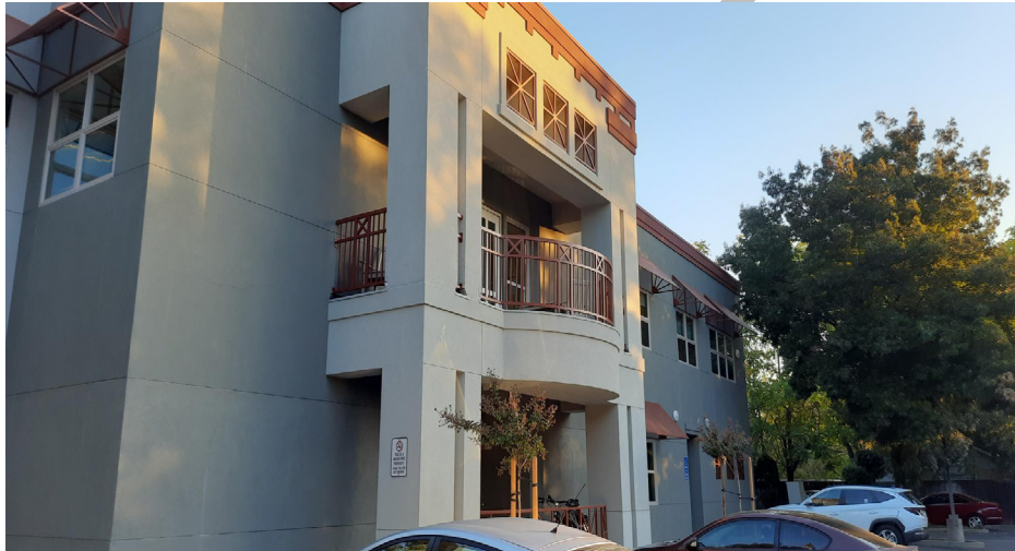
Figure 2: Office of the Shasta Regional Transportation Agency
