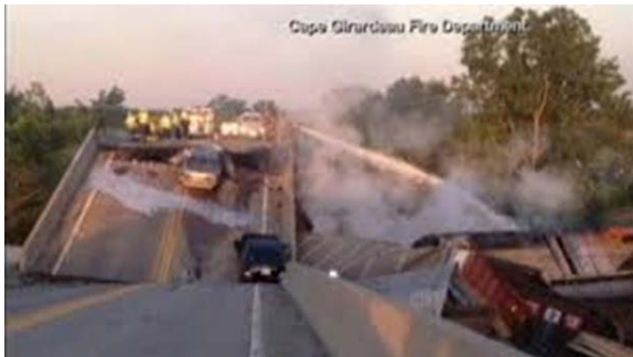
Figure 1 Union Pacific train derailed highway structure collapse, Missouri, 2013.
