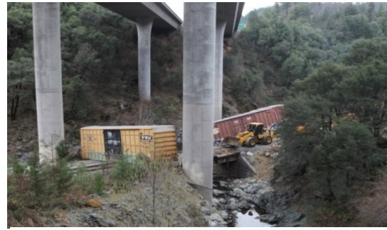
Figure 2 Union Pacific Train Derailment at I-5 in Shasta County, 2014.
