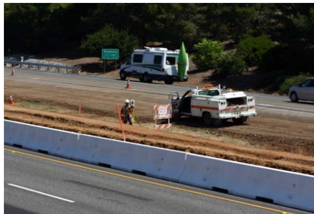
South Redding Six-Lane Construction, 2011.
